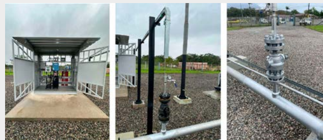
Figure 12 – The Chromatograph Installation in Joinville
