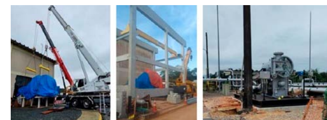
Figure 24 – Removal of the motor-compressor from Araucária/PR, assembly of the work area and installation of the filter unit in Biguaçu/SC
