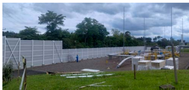
Figure 23– Installation of the noise barrier at the Siderópolis/SC Compression Station
