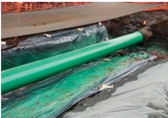
Figure 14 – Recoating process conducted at the Compression Station in Campo Grande/MS
