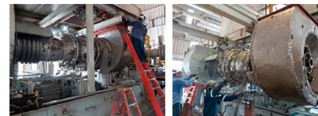
Figure 19 – Turbine substitution at the Compression Station in Corumbá/MS
