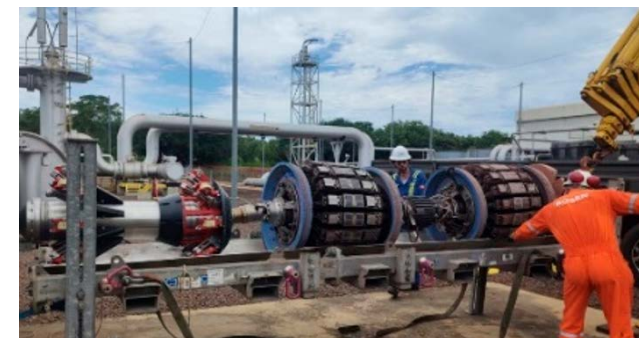
Figure 15 – PIG instrumented inspection process
